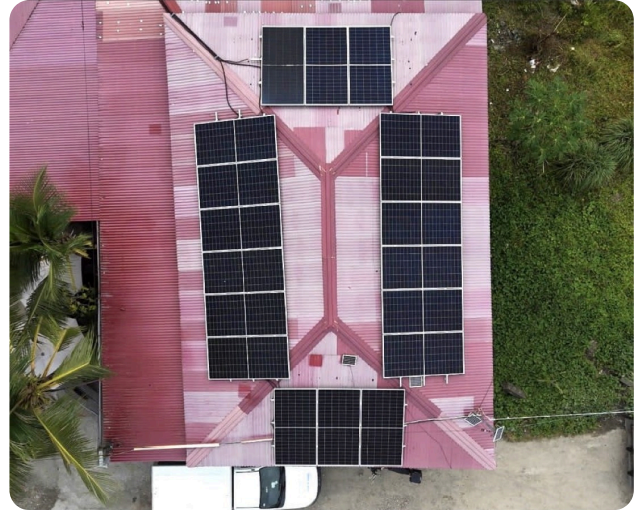
CONTHEA INN AND RESTAURANT. 10 KWP HYBRID, 2 × 280 AH STORAGE, HOSPITALITY.
