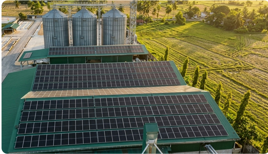
THE 350 KWP ROOFTOP ARRAY THAT STARTED IT ALL, AT THE VM AGBAYANI RICEMILL IN ORIENTAL MINDORO.
